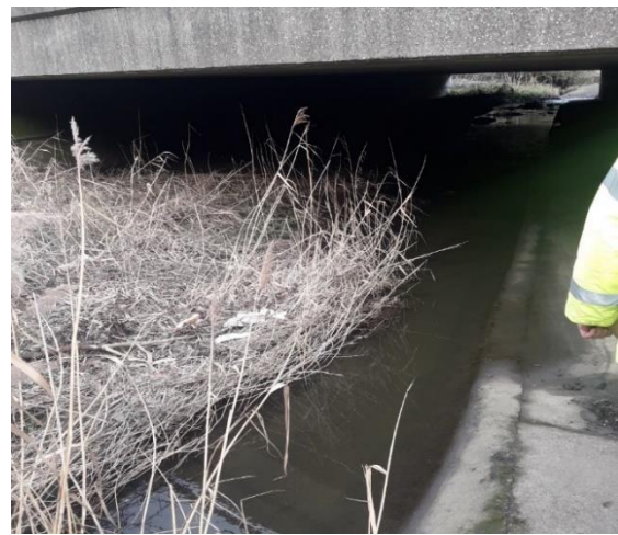
Mardyke West – existing culvert beneath the M25. Date: October 2017
